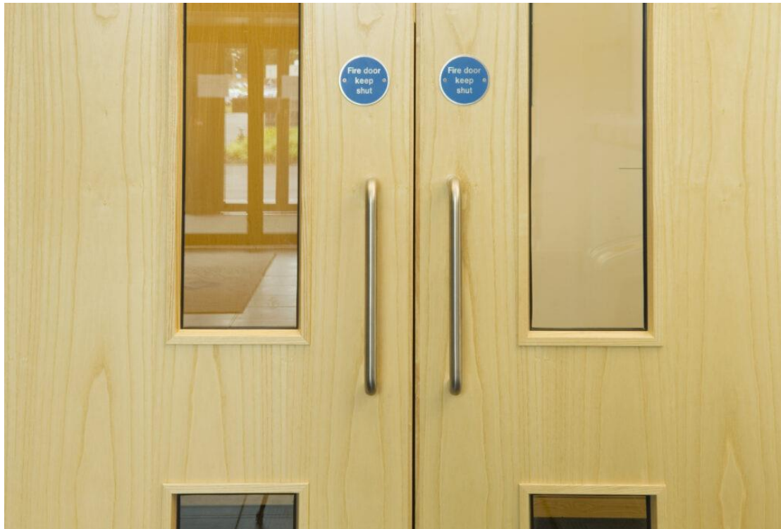
Above - An example of Fire doors with blue labeling system.
